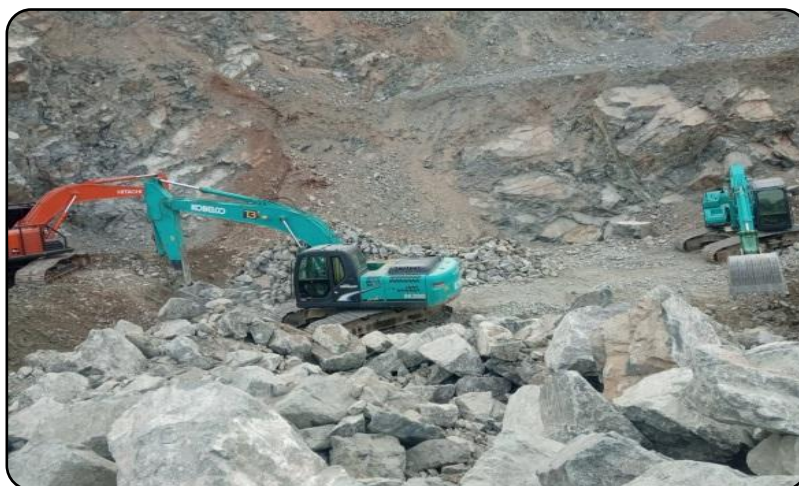
Figure 3: Quarry and Jetty Conditions
